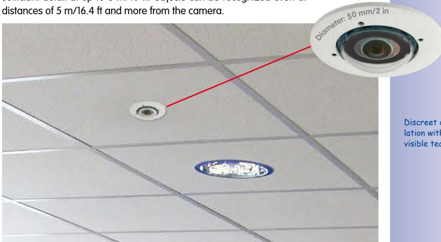
Discreet ceiling installation with minimally visible technology
